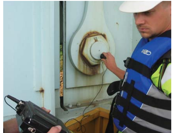
Bridge pin UT inspection.
