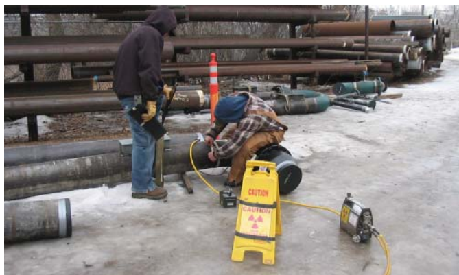
RT on 10 inch pipe weld.
